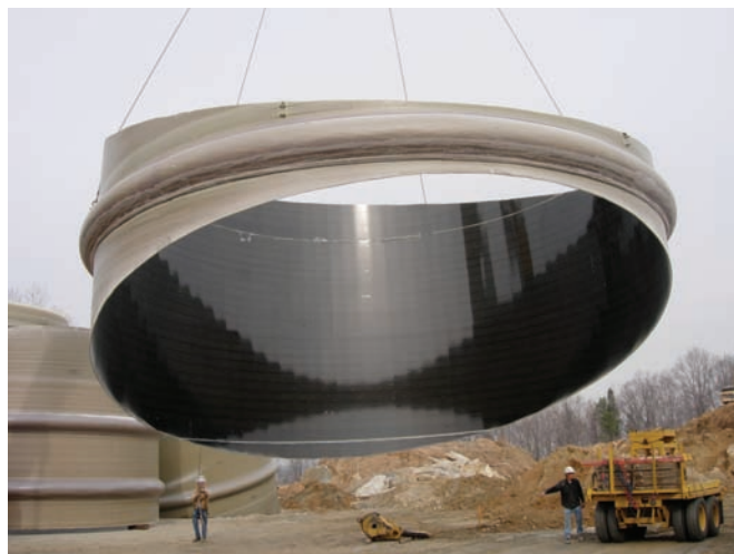
Section of composite flue stack with Hollingsworth & Vose carbon fiber-based surfacing veil visible. Photo courtesy of Ershigs, Inc.
